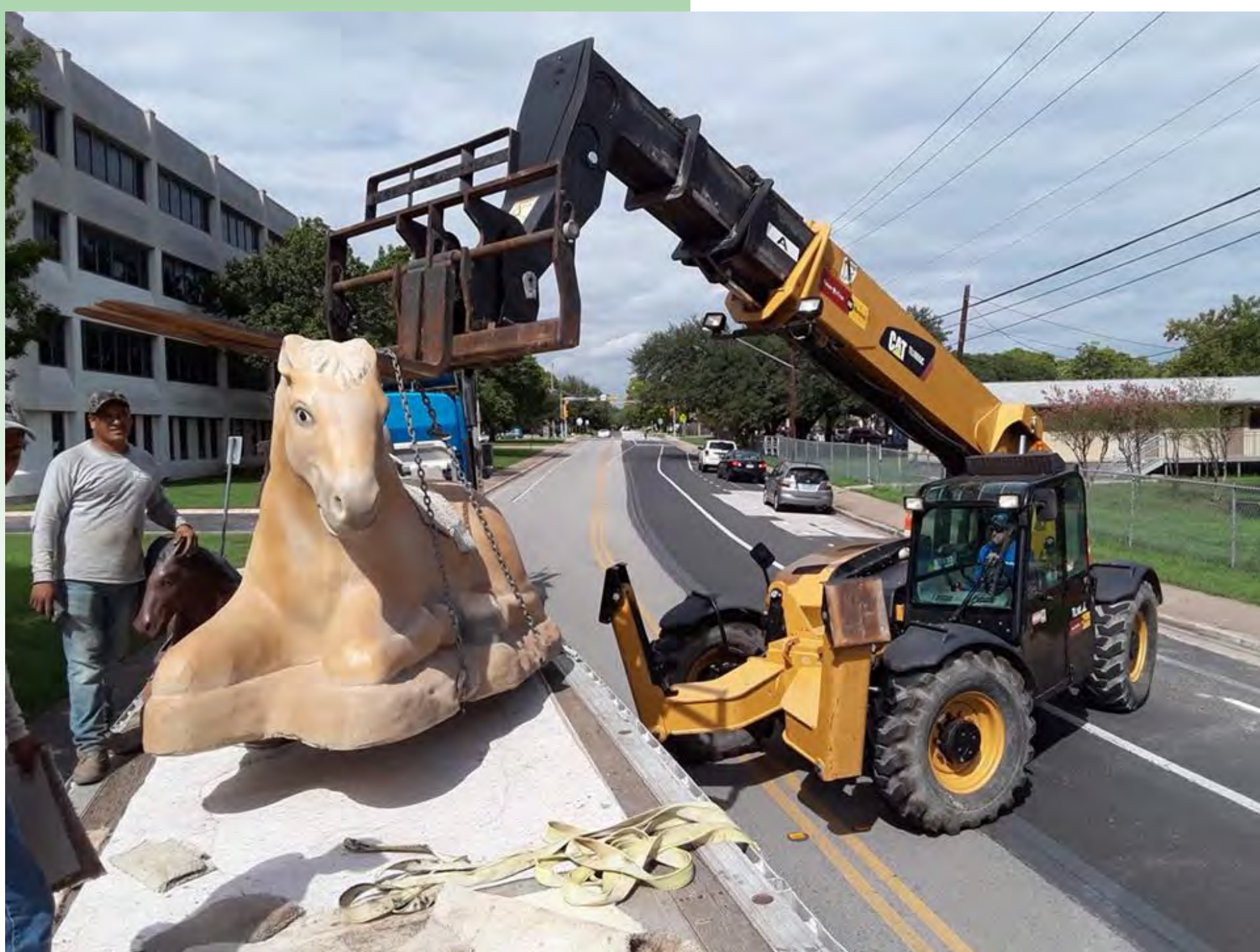
Playground Installation Denton, TX
