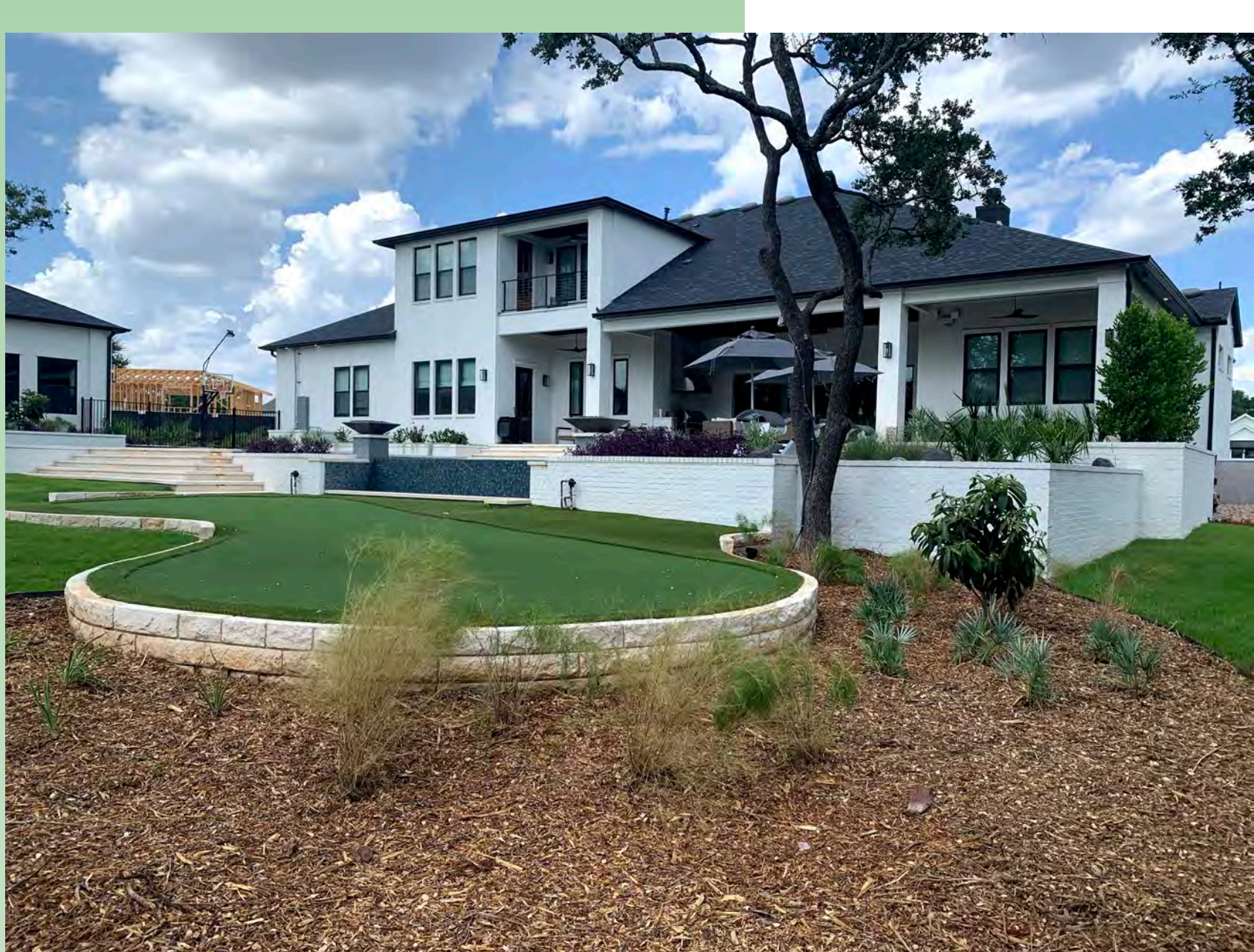
Backyard install Denton, TX
