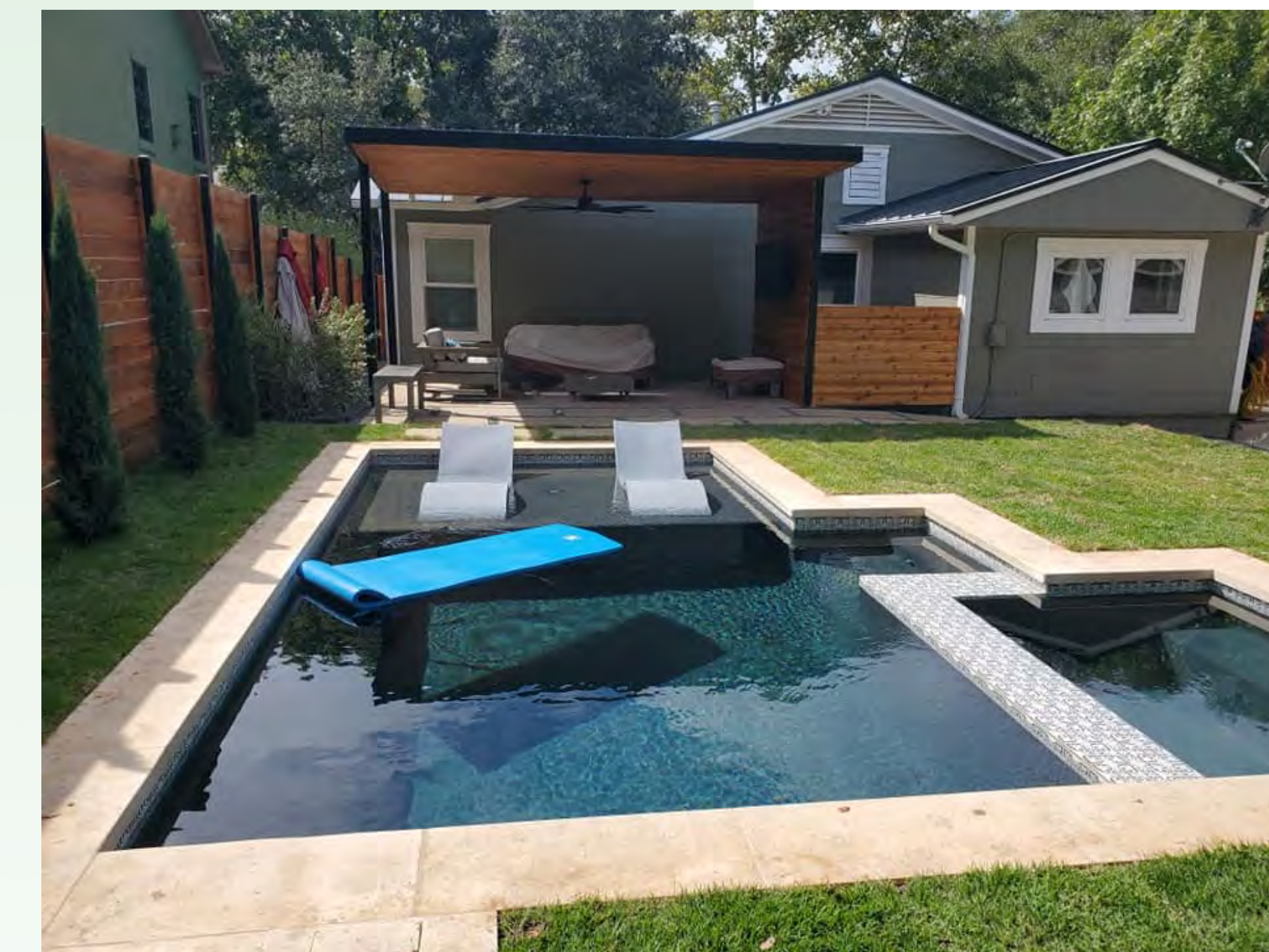
Backyard install Denton, TX
